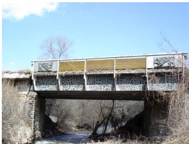
Figure 1 – Ginzi Highway GFRP- Bridge, Bulgaria
